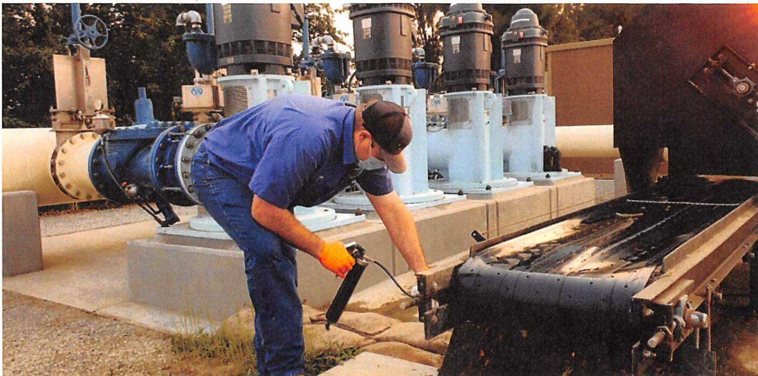
Byron-Bethany Irrigation District - Tony Papini conducting maintenance at Pump Station #4.
